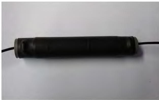
Now apply the heat shrink tubing and heat evenly until the heat shrink fits nicely.
